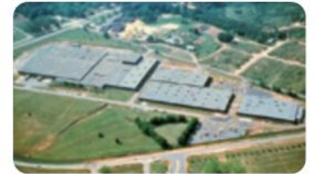
YKK (U.S.A.) Inc. Macon Plant
