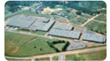
YKK (U.S.A.) Inc. Macon Plant
